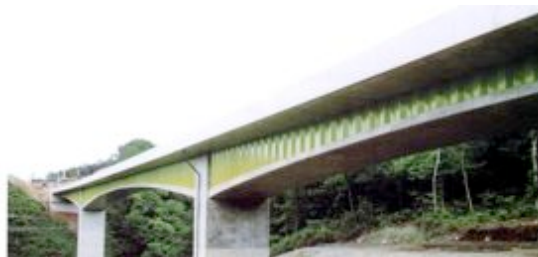
External post-tensioned bridge
