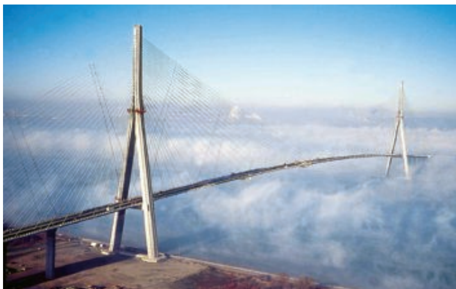
The Normandy Bridge (photo Bouygues Campeon Bernard Group - Vinci)
