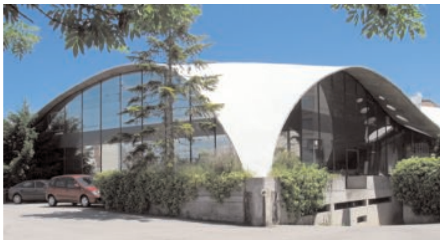
Shell structure designed and built by Heinz Isler for Sicli SA, Geneva, Switzerland
