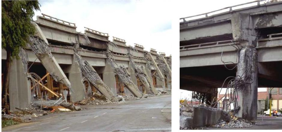
Fig. 10-8: Sliding shear at top columns of the Cypress viaduct in the 1989 Loma Prieta earthquake (after NISEE, 2000).
