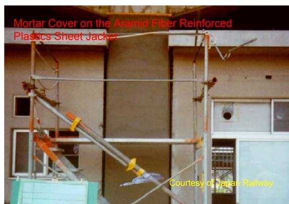
Fig. 11-30: Aramid fiber reinforced plastics jacketing for a railway viaduct [courtesy of JR Research Institute]
