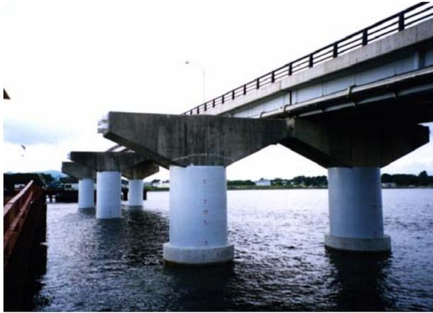
Fig. 11-31: Piers retrofitted by aramid fiber sheet [Kato et al. (2001)]
