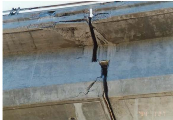
Fig. 11-61: Damage of intermediate joint due to pounding (1994 Northridge earthquake)
