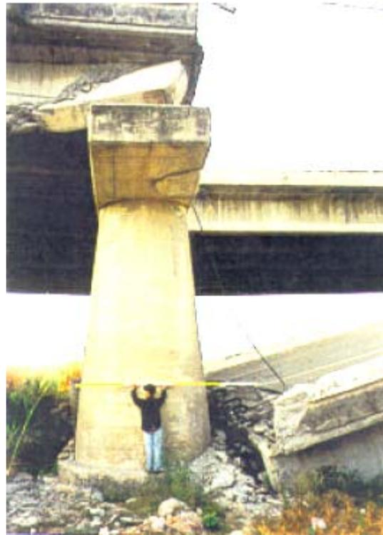
Fig. 8-2: Wushi Bridge - span collapse due to longitudinal movement at pier P2N
