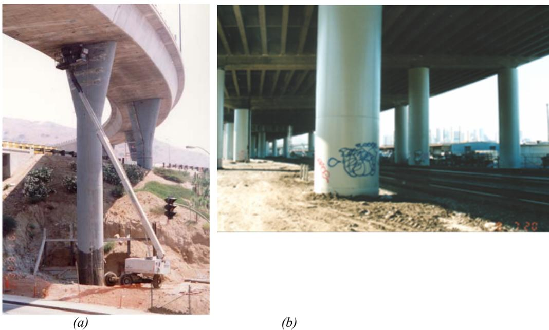
Fig. 11-2: Steel jacket retrofit of columns: (a) Los Angeles, and (b) San Francisco
