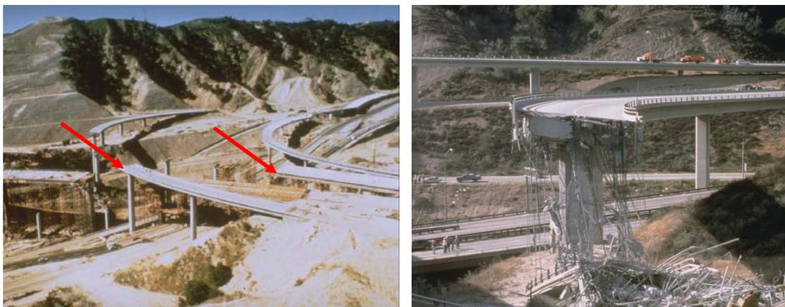
Figure 10-1: Span collapses at the Golden State-Antelope Valley interchange collectors during the 1971 San Fernando (left) and the 1994 Northridge (right) earthquakes (courtesy of USGS).
