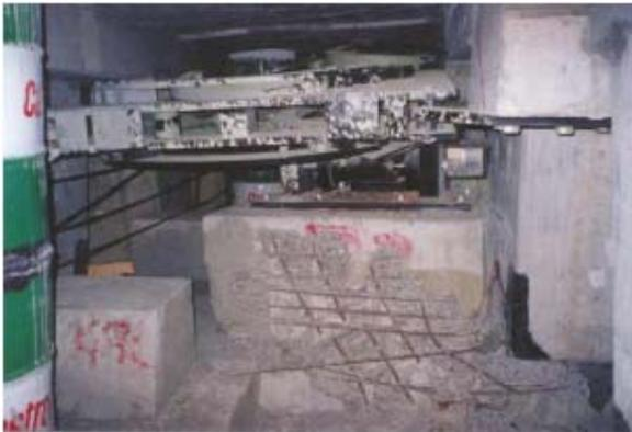
*Fig. 8-7: Bolu Viaduct - failure of an EDU*
