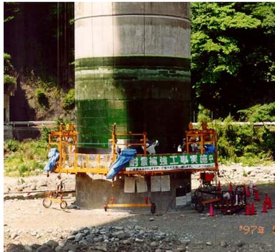
Fig. 11-27: Carbon fiber sheet jacketing of hollow reinforced concrete columns, Sakawa-gawa bridge, Tomei expressway; (a) Retrofitted east- and west-bound bridge, and (b) Wrapping of carbon fiber sheets [Ogata et al. (1999), Osada et al. (1999)]
