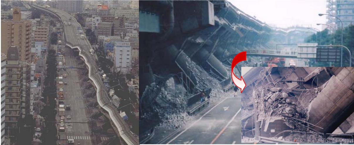
*Fig. 10-5: Flexural failure above column base of columns of the Hanshin expressway, due to premature termination of longitudinal reinforcement and inadequate confinement in the 1995 Kobe earthquake (courtesy of Kawashima).*
