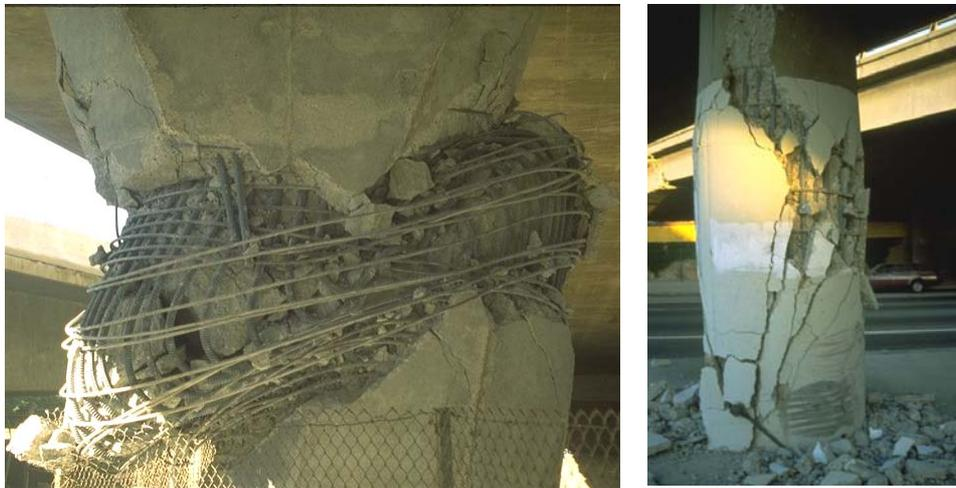
*Fig. 10-6: Shear failure within (left) and outside (right) the plastic hinge region in San Fernando Mission Blvd-Gothic Avenue Bridge and I-10 Freeway at Venice Blvd, respectively, during the 1994 Northridge earthquake (after NISEE, 2000).*
