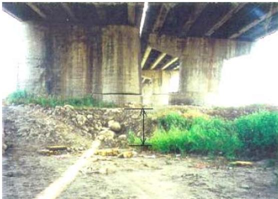
Fig. 8-1: Wushi Bridge - fault movement between piers 2 and 3
