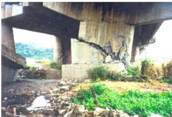
Fig. 8-3: Wushi Bridge - shear failure of pier P2S
