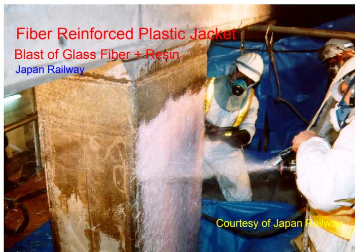
Fig. 11-34: Glass fiber jacking (courtesy of JR Research Institute)
