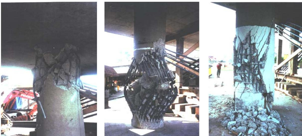
*Fig. 10-7: Different shear damage patterns for RC piers at the under-crossing of the Santa-Monica Interstate during the 1994 Northridge earthquake: Piers # 5 with inadequate detailing for plastic hinge (left), Piers # 6 with symmetric buckling (middle) and Pier # 8 with typical shear failure (right) (after Broderick et al., 1994).*
