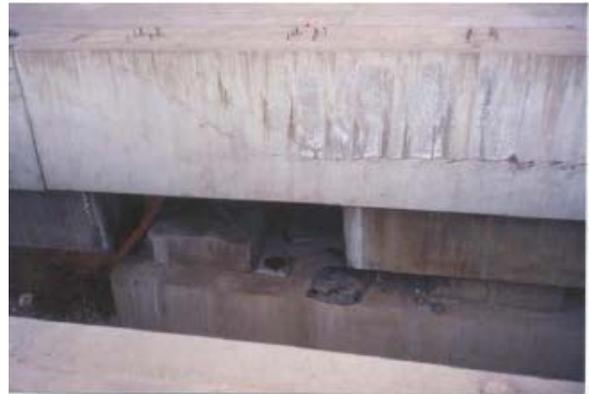
*Fig. 8-8: Bolu Viaduct - unseating of beam end at pier cap*
