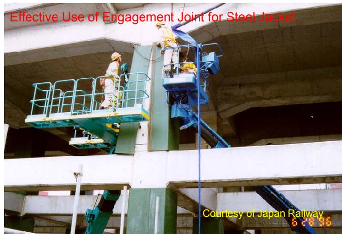
Fig. 11-14: Effective use of engagement joint for retrofit at a railway viaduct (JR Research Institute)
