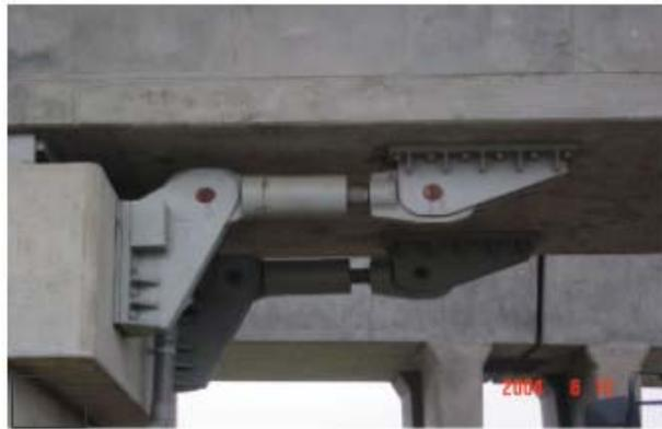
Fig. 6-25: Representation of the viscous damper units in the Rion-Antirion bridge (<http://www.gefyra.gr>) (left), example of viscous dampers application to a bridge located at Yen-Chou in Taiwan (Hwang and Tseng, 2005) (right).
