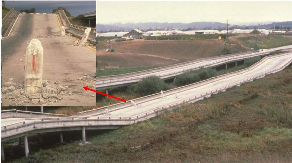
*Fig. 10-2: Punching of piles through the road bed of the State Route 1, Watsonville area, span during the 1989 Loma Prieta earthquake (after NISEE, 2000).*
