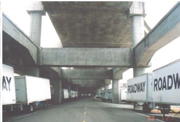
Fig. 11-46: Retrofit of San Francisco double-deck viaducts using edge link beams: (a) as-built viaduct, (b) proof test model, (c) proof test, (d) column damage in the proof test, (d) retrofit, and (e) edge beams [(a)-(d): Priestley, Seible and Calvi (1996)]
