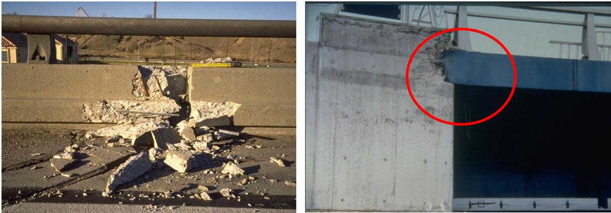
*Fig. 10-3: Pounding damage: between adjacent spans at the Interstate-5 at Santa Clara River in Los Angeles County during the 1994 Northridge earthquake (left) and at the abutment of a bridge near Nishinomiya Port in the 1995 Kobe earthquake (after NISEE, 2000).*
