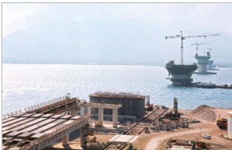
*Fig. 5-16: View of the Antirion access viaduct during construction (see pile cap above ground surface)*
