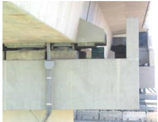
*Fig. 8-16: Piers with extended seating length and special bearings*
