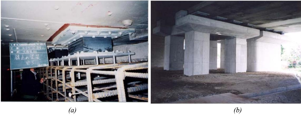
Fig. 11-67: Seismic retrofit using isolation: (a) installation of lead rubber bearings and sliding bearings, and (b) after retrofit (courtesy of Japan Highway Public Corporation)
