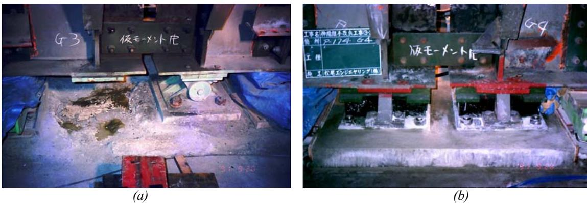
Fig. 11-68: Connection of decks and retrofit: (a) removal of existing steel bearings, and (b) set of new lead rubber bearing (courtesy of Hanshin Expressway Public Corporation)
